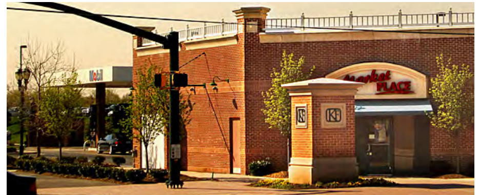
A gas station with a convenience store in front and pumps in the back (left of the photo) creating a more amenable environment for pedestrians (Source: Brett VA, Flickr).
