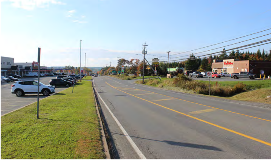
Right-of-way along Trunk 7
